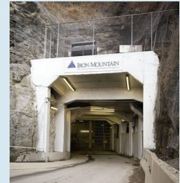
Entrance to data center.
